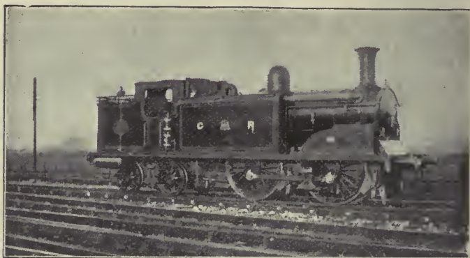
FIG 125.—MOINTOSH'S 5FT. 9IN. CONDENSING TANK ENGINE, CALEDONIAN RAILWAY
