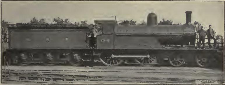
FIG. 136.—“No. 1312,” ONE OF MR. IVATT’S (1073) SMALLER CLASS OF 4-COUPLED BOGIE ENGINES FOR THE GREAT NORTHERN RAILWAY.
